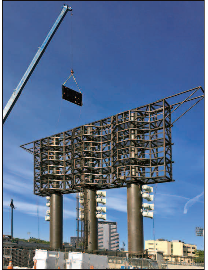
A crane lifted jumbo screen components onto the larger frame as part of the installation process. Photos by Justin Purdy
